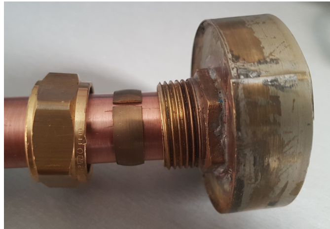
Fitting a choke to the 22mm CU-pipe.
